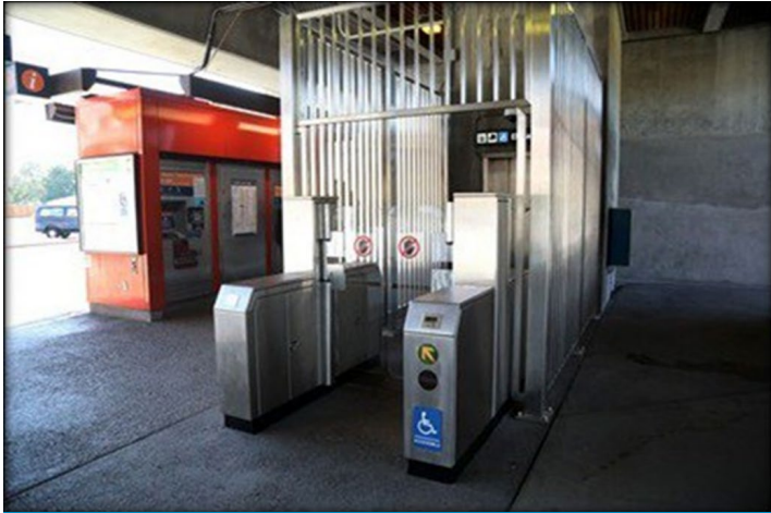
CONCORD (Completed Oct 2020)
