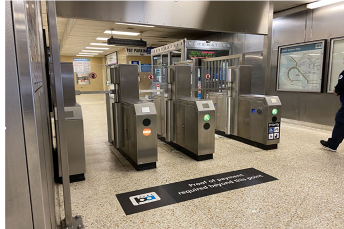
ROCKRIDGE ARRAY 1 (Completed Aug 2021)
