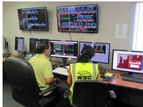
Systems Integration testing is underway.
